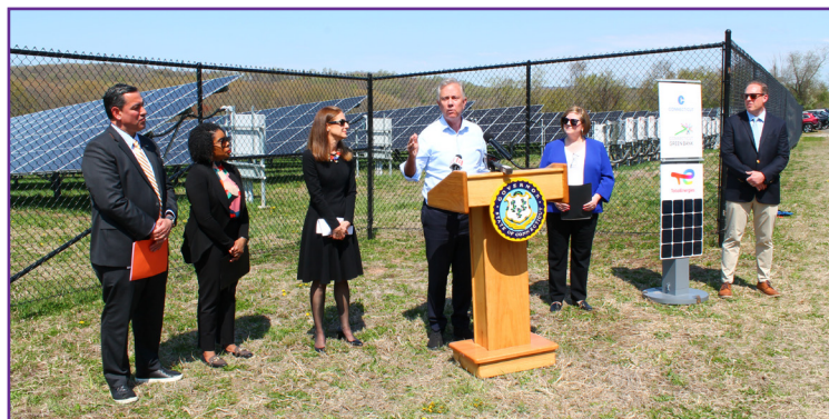
Governor Lamont addressed the crowd gathered at Cheshire Correctional Institution with the 2.4 megawatt solar system in the background. Also pictured, from left to right, are Bryan Garcia, President and CEO of the Green Bank, DOC Deputy Commissioner Sharonda Carlos Lt. Gov. Susan Bysiewicz, DAS Commissioner Michelle Gilman, and Alex Sarly, Associate Director, Development, TotalEnergies.
